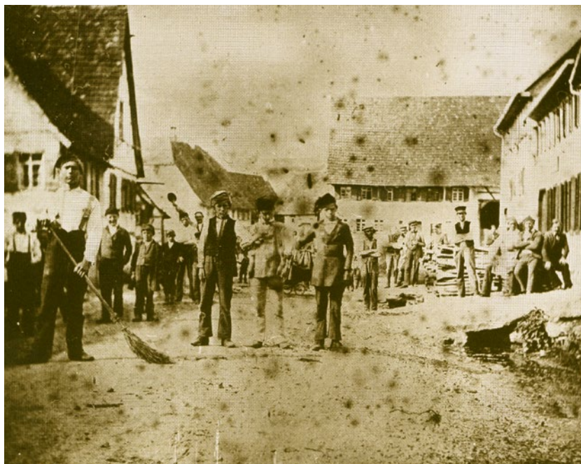
Probably the oldest photo of Wilhelmstrasse, with mould stains.
